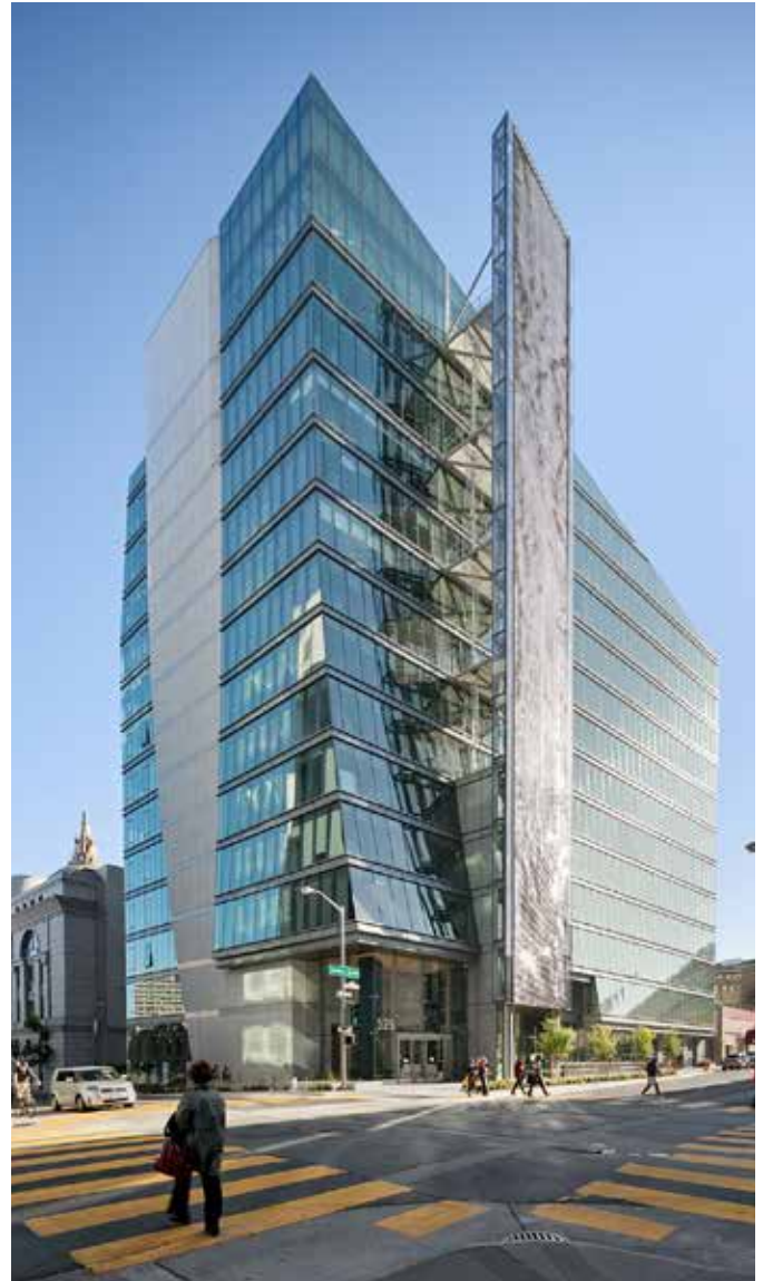
San Francisco Public Utilities Commission Headquarters, San Francisco, CA
