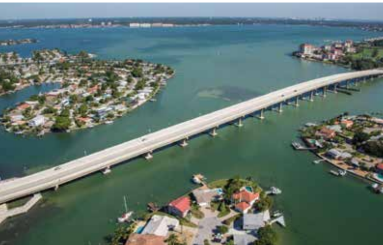
Pinellas Bayway Bridge, St. Petersburg, FL
