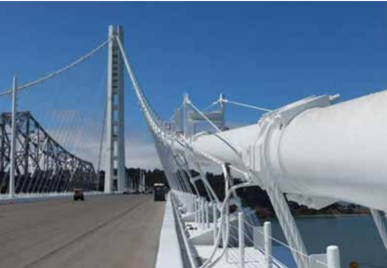
San Francisco–Oakland Bay Bridge, Eastern Span, San Francisco, CA
