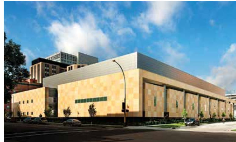
Richard O. Jacobson Building, Rochester, MN (photo courtesy ©Dean Riggott Photography)
