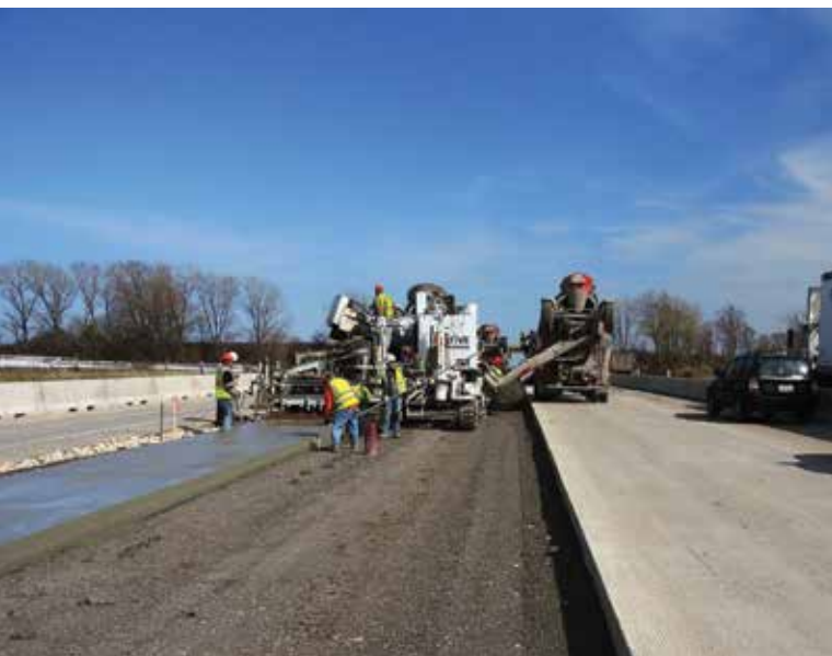
Illinois Tollway I-90 Westbound Mainline Paving Upgrades, Rockford-Elgin, IL
