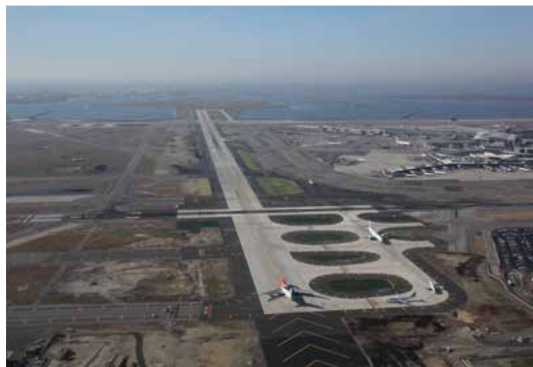
JFK International Airport – Runway 4L-22R Reconstruction, New York, NY
