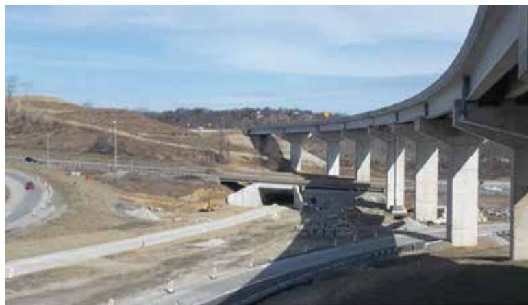
I-79/I-70 South Junction Interchange, Washington County, PA
