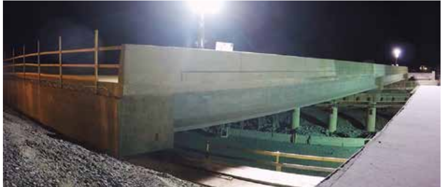
ODOT Rt. 6 bridge slide
