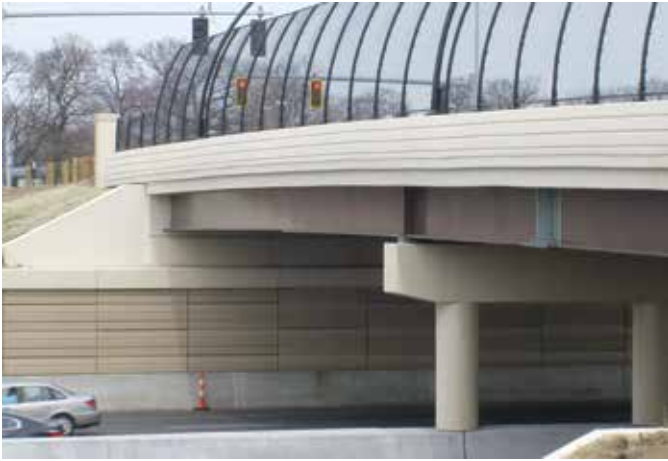
Ohio Department of Transportation Project 10-0281 ProMedica Bridge Deck, Toledo, OH
