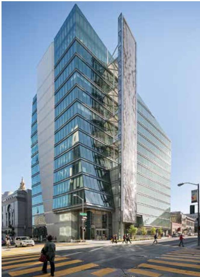
San Francisco Public Utilities Commission Headquarters, San Francisco, CA
