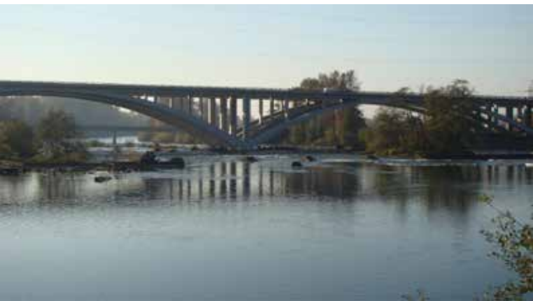
Willamette River Bridge, Eugene, OR
