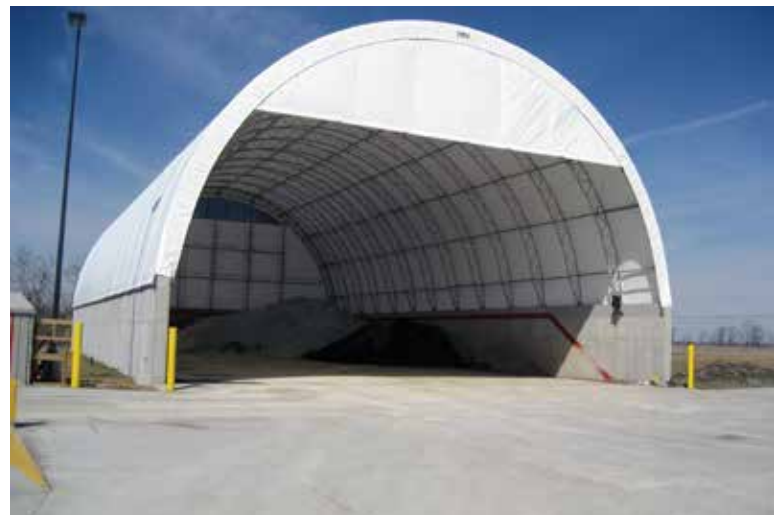
Ohio Department of Transportation Jefferson County Maintenance Facility, Wintersville, OH
