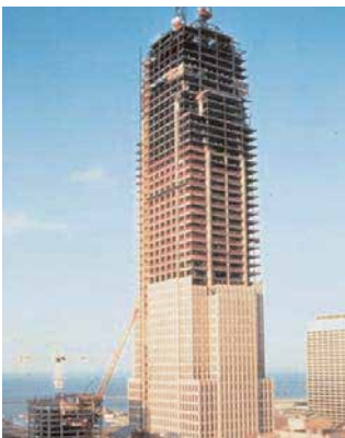
Structural concrete in the Key Tower (formerly Society Tower) in Cleveland achieved over 13,000 psi using a portland-slag cement-silica fume ternary mixture.
