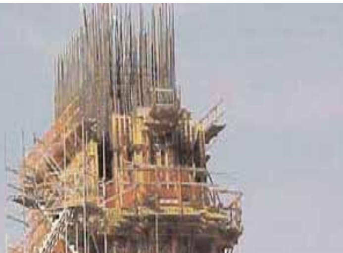
Figure 1: NRG Stadium (NFL) in Houston, TX, which opened in 2002, used a portland-slag cement-fly ash mixture to achieve both high strength and low heat of hydration in its four massive “super columns,” supporting the retractable roof.
